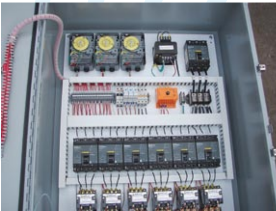
LIFT STATION CONTROL PANEL FOR WASTE WATER TREATMENT PROJECT
